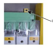
**ATICS-2-DIO**: Now use the screwdriver to pull the upper yellow slide lock (D) upwards and remove the ATICS®.
